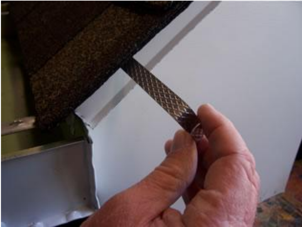
Lift on edge of shingle
